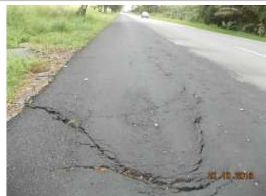
V-shape cracks due to horizontal tensile strain
