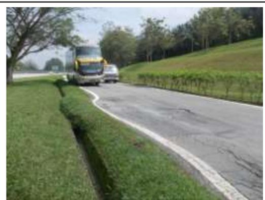
Vertical deformation in cut ground
