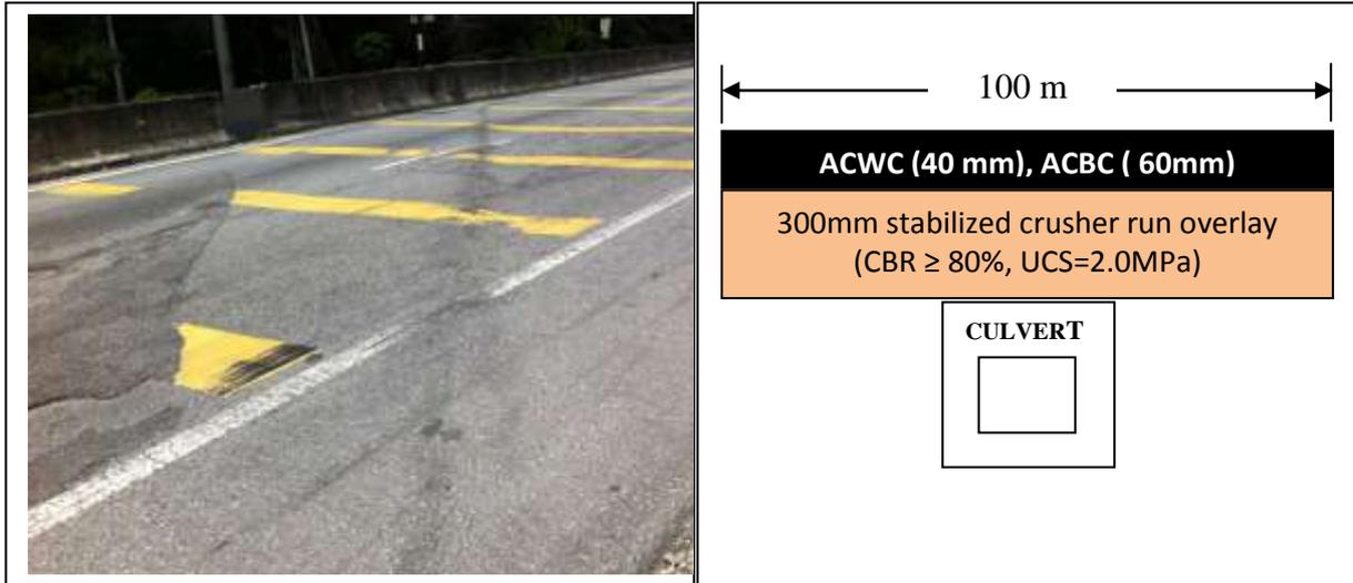
Photo 4: Culvert ‘hump’ at culvert crossing.
