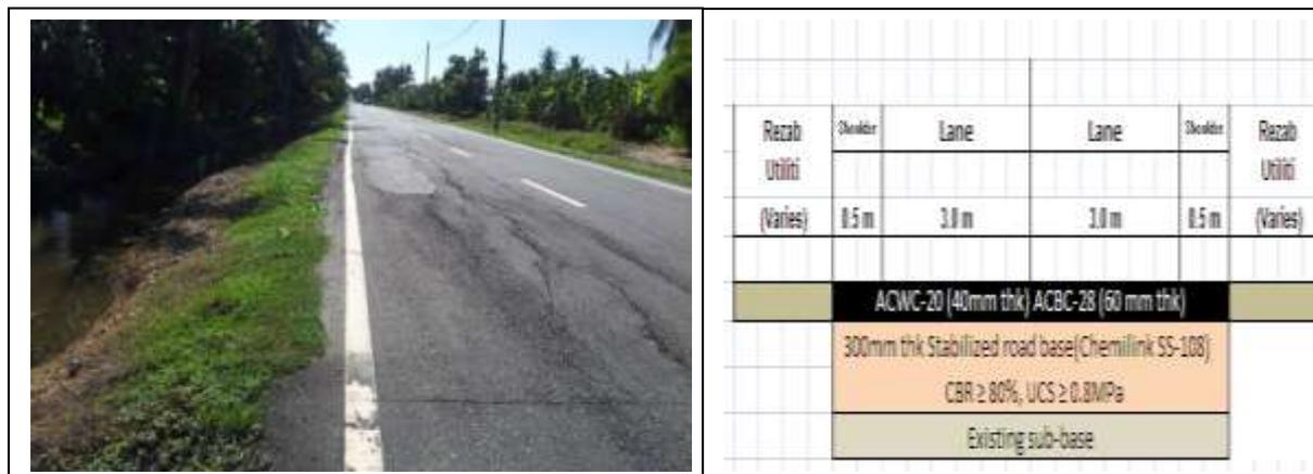
Photo 5: Road keep ‘sinking’ with no end.
