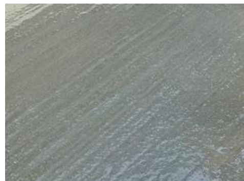
Finished wet surface
