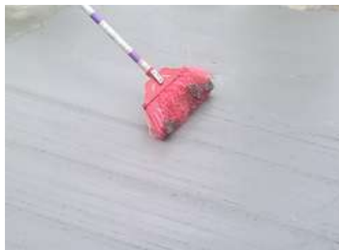
Brooming the surface
