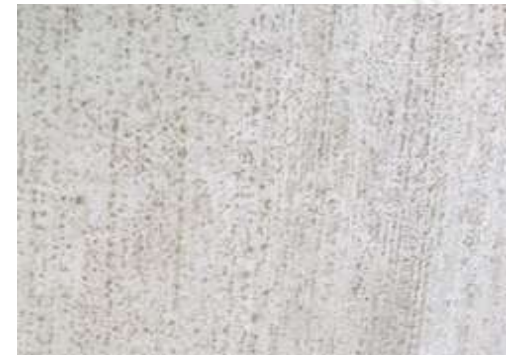
Finished dry surface
