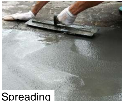
Substrate Preparation
