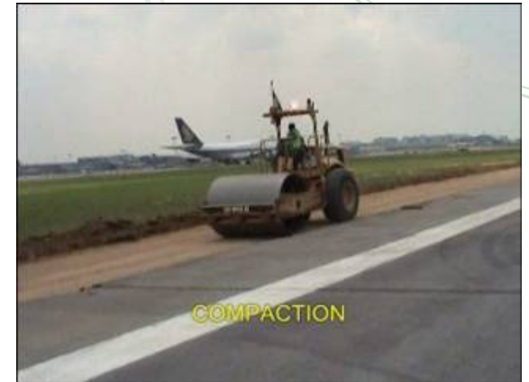
c) Compaction
