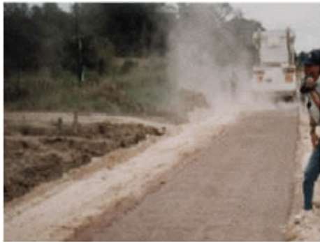
Mechanical Spreading
