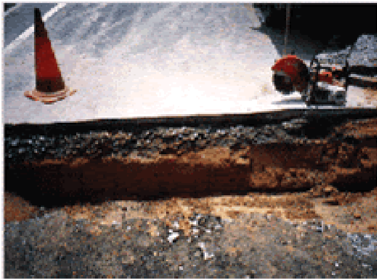
a) Opened Road Cross Section
