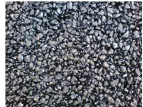
Finished Surface of Porous Asphalt Concrete
