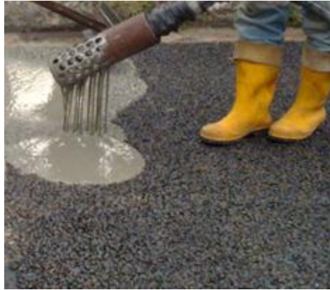
Filling Cement Mortar into Porous Asphalt Concrete
