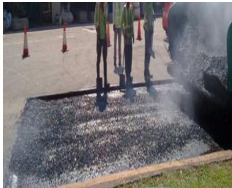
Laying Porous Asphalt Concrete
