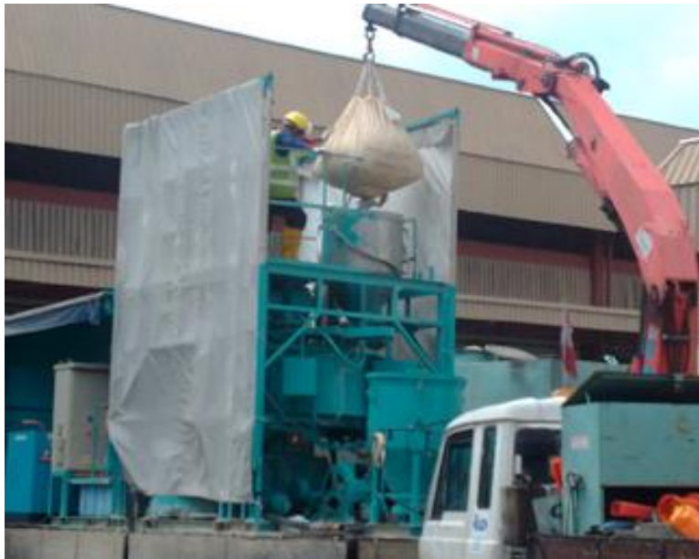
Loading Polymer Modified Mortar Into Mixer
