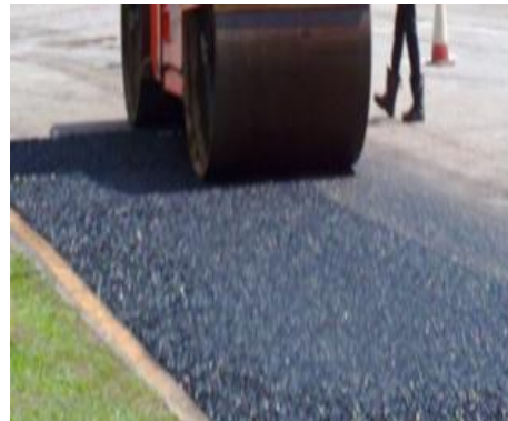
Compacting Porous Asphalt Concrete
