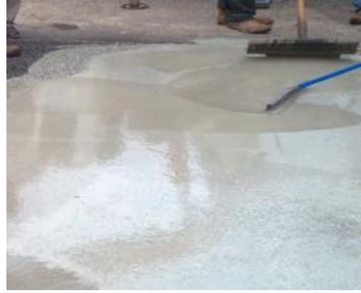
Spreading Cement Mortar
