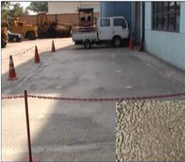
(a) Semi-Rigid Pavement after Hardened
