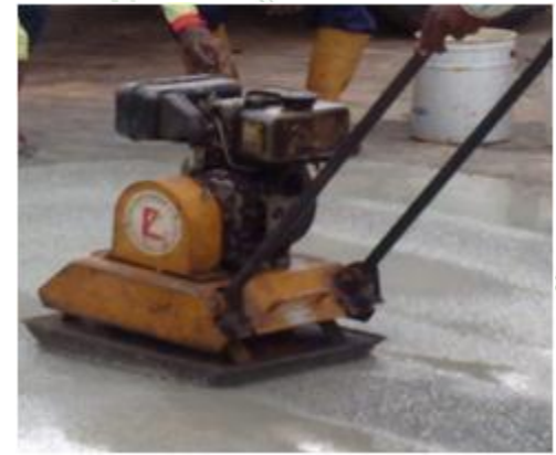
(b) Leveling and Vibration (if needed)
