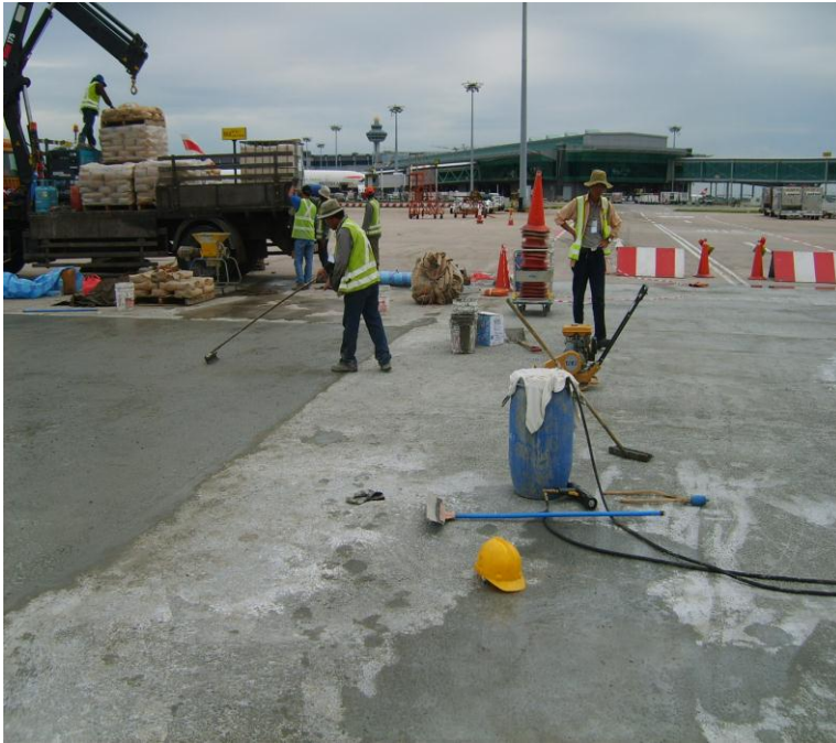
Semi-rigid Pavement for Airport Aprons Construction in Progress
