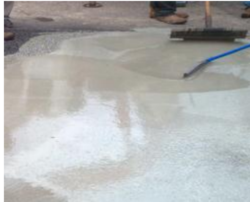
(b) Leveling and Vibration (if needed)
