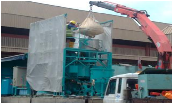
(a) Loading the Mortar into Big Mixer
