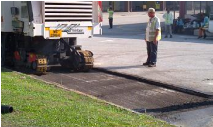
(a) Milling of Existing AC Surface
