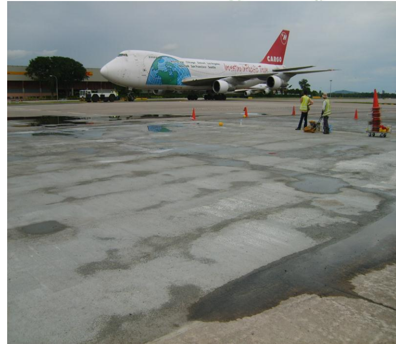
Semi-rigid Pavement for Airport Aprons Construction in Progress
