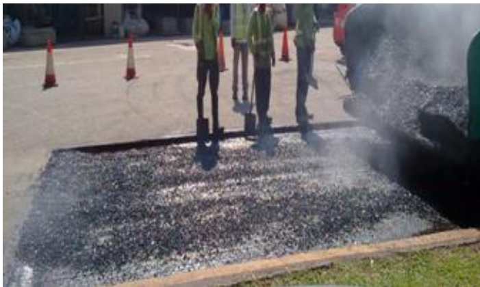
(c) Laying PAC to Design Thickness
