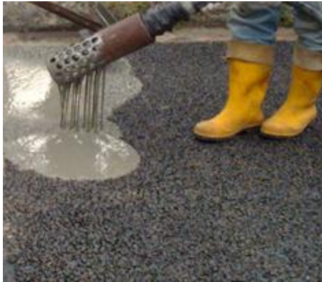
(a) Filling the Mortar into PAC
