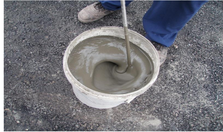
(d) Mixing the Mortar with Water
