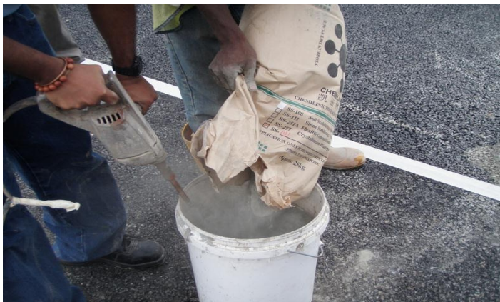
(c) Loading the Mortar into Small Mixer
