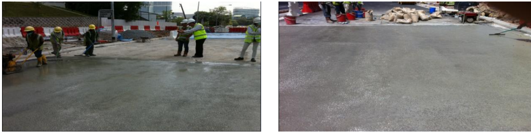
Fig. 8 Semi-rigid pavement system in construction in city area
