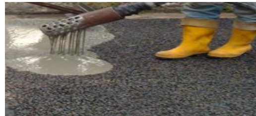
Fig. 3b Grouting of the mortar
