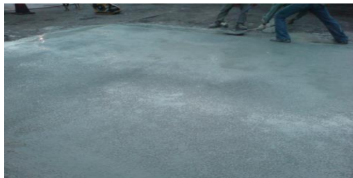
Fig. 7a Construction in progress
