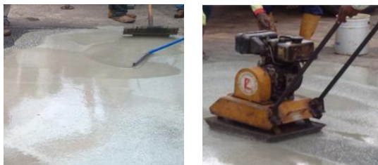
Fig. 3c Levelling and vibration (if needed)
