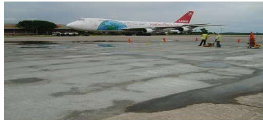
Fig. 5 Semi-rigid pavement for airport aprons construction in progress
