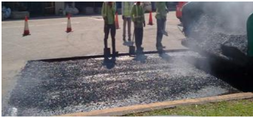
Fig. 2c Laying PAC to design thickness
