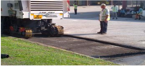
Fig. 2a Milling of existing AC surface
