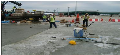
Fig. 5 Semi-rigid pavement for airport aprons construction in progress
