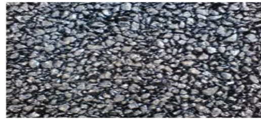
Fig. 2d PAC surface after compaction (air voids 25-30%)
