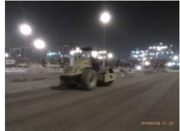
Step 3: Compaction
