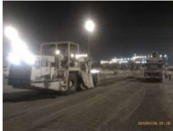
Step 2: In-Situ Mixing
