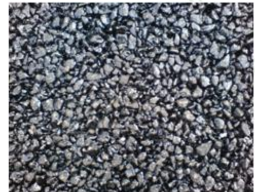
Finished Surface of Porous Asphalt Concrete
