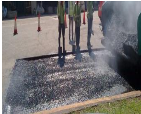
Laying Porous Asphalt Concrete
