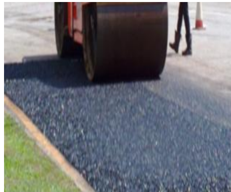
Compacting Porous Asphalt Concrete
