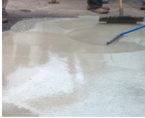
Spreading Cement Mortar
