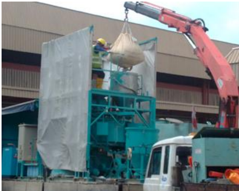
Loading Polymer Modified Mortar into Mixer
