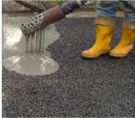
Filling Cement Mortar into Porous Asphalt Concrete
