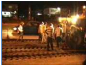
a) Road Partially Closed during Night for Maintenance
