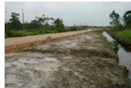
b) Sub-Grade Conditions
