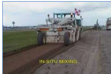
b) In-situ Mixing
