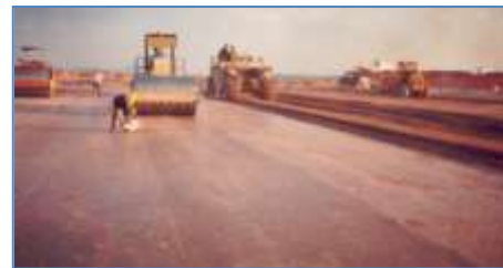
b) In-Situ Mixing and Compaction
