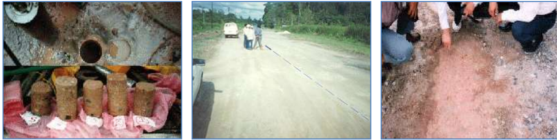
a) Stabilized Soil Samples
