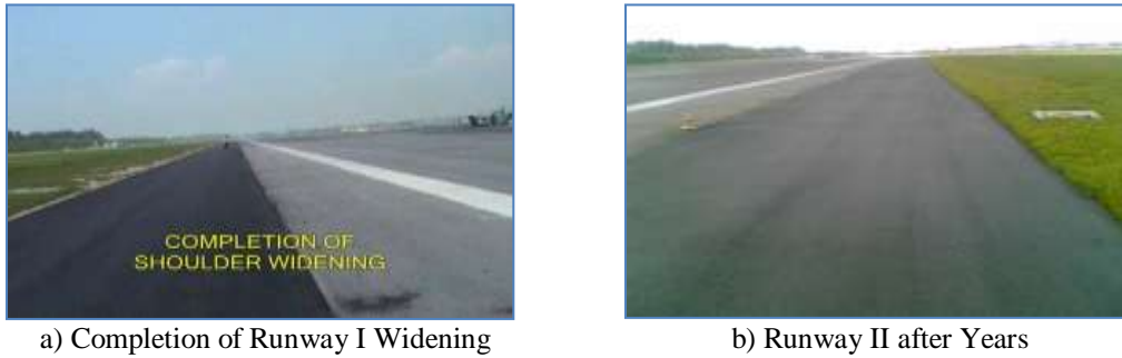
Photo. 2. Runways Widening in Singapore Airport
