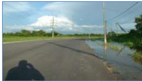
Photo. 10. A Stabilized Road at Low-Lying Area (2004)
