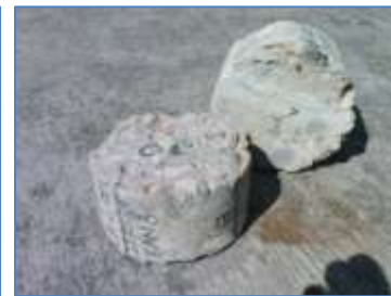
c) Cored Samples with Recycled In-Situ Materials
