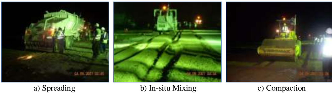
Photo. 3. Soil Stabilization in Senai Airport
