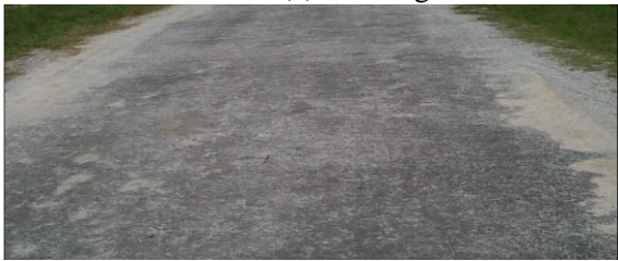
(b) Road condition after 7 months with minor chip seal defects (photos taken at August 2010)
