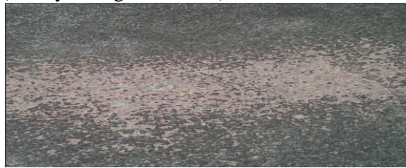
(b) Road condition after 7 months with minor chip seal defects (photos taken at August 2010)
