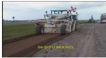
In-situ Mixing (Stabilizer)
