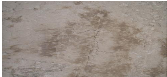
(a) Existing road condition (Muddy and Shrinkage cracking)
