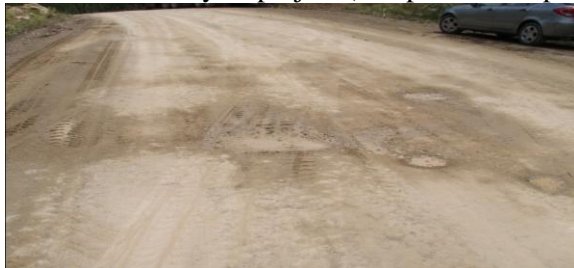
(a) Existing road condition (Muddy and Shrinkage cracking)
