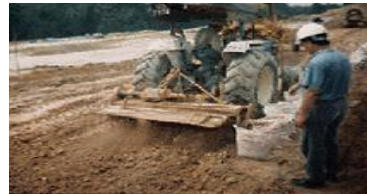
In-situ Mixing (Rotovator)
