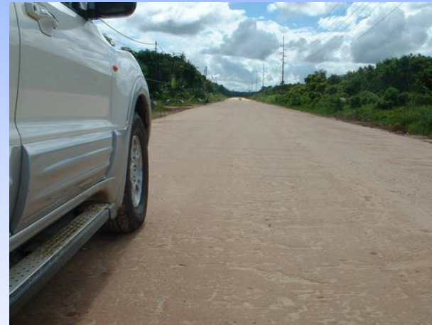
Mixture after Compaction
