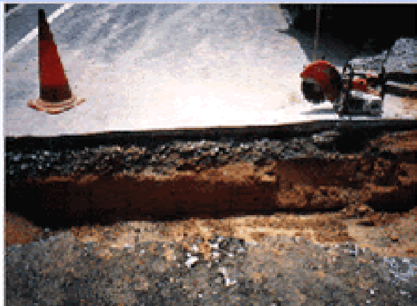
a. Opened road cross section
