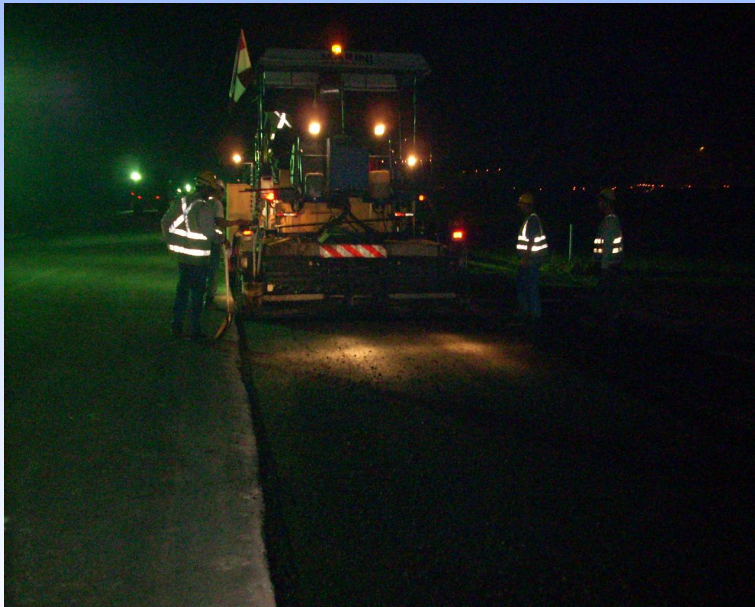
e) Paving Asphalt Concrete
