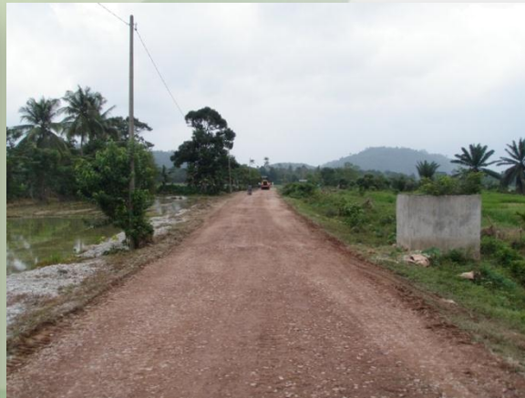
After Chemilink Stabilization
