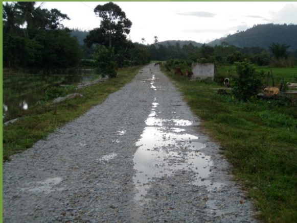
Before Chemilink Stabilization
