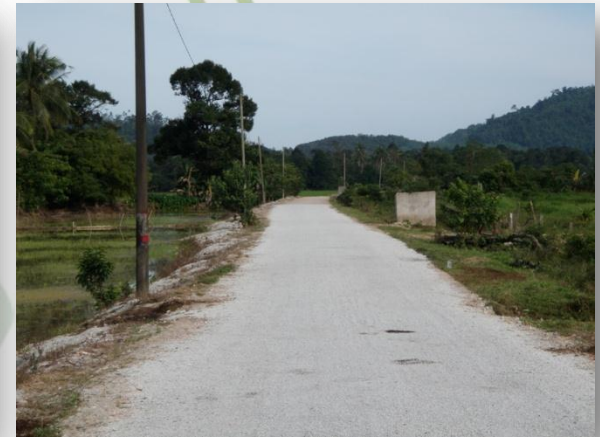
Chip Seal Surface
