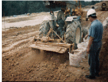
Mixing by Rotorvator
