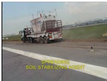
Mechanical Spreading
