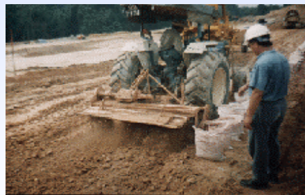
Mixing by Rotorvator
