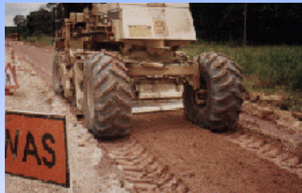
Mixing by Stabilizer
