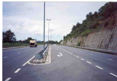
Photo. 2. Jalan Tutong Widening, Phase II (4 years later)
