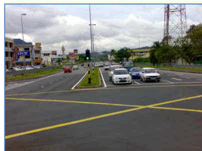
b) Road after 10-Year Completion
