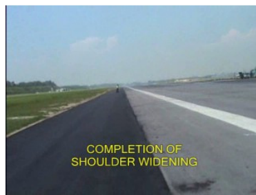
Photo. 6. Completion of Runway Widening in Changi Airport
