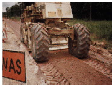
Mixing by Stabilizer
