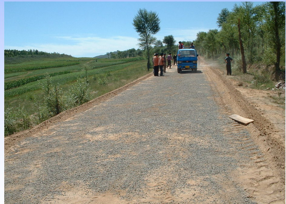
Spreading chips on the surface
