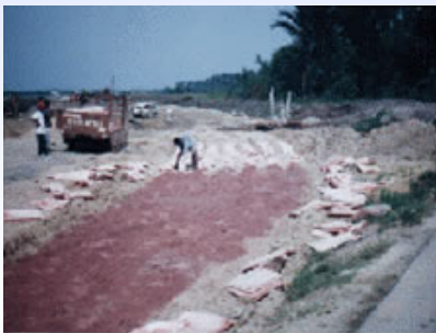
Manual Spreading
