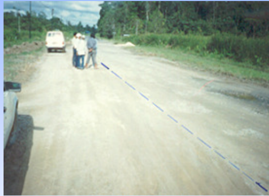
b) Stabilized Road (on the left) vs. Old Road
