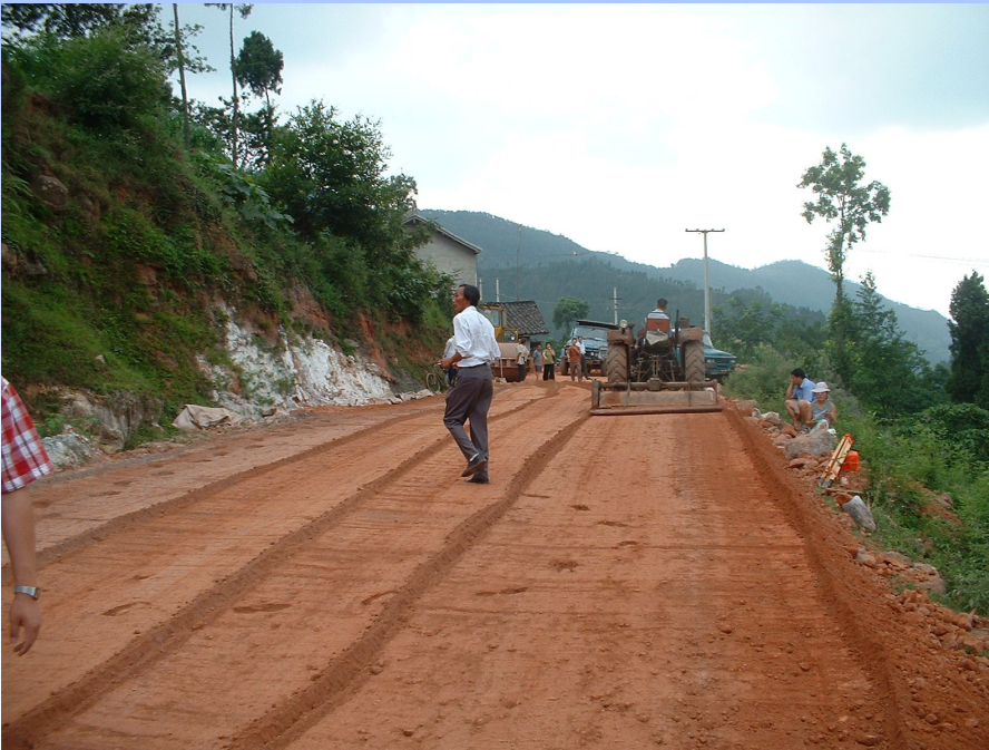
Mixing by Rotorvator
