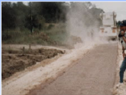
Mechanical Spreading
