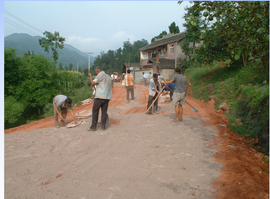
Manually Spreading
