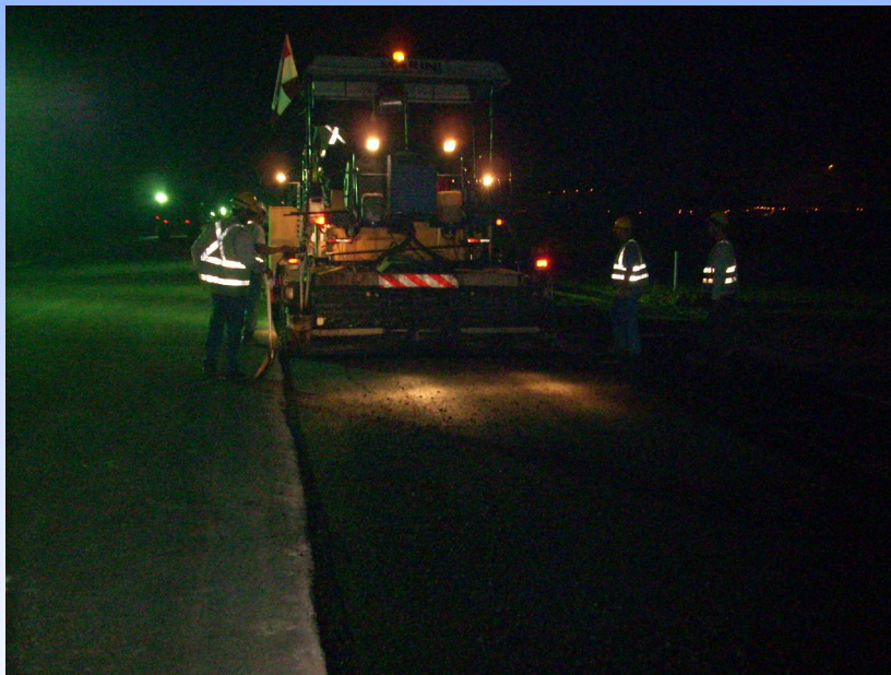
e) Paving Asphalt Concrete
