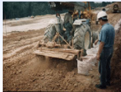
Mixing by Rotorvator
