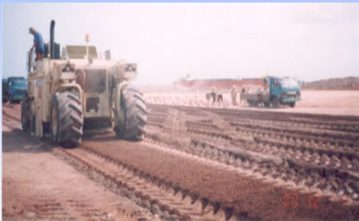
a) Manual Spreading and Mechanical Mixing
