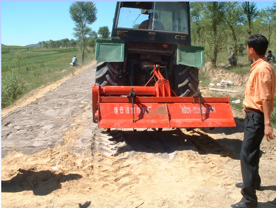
Mixing by Rotorvator
