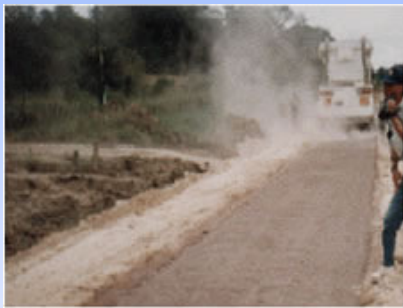
Mechanical Spreading
