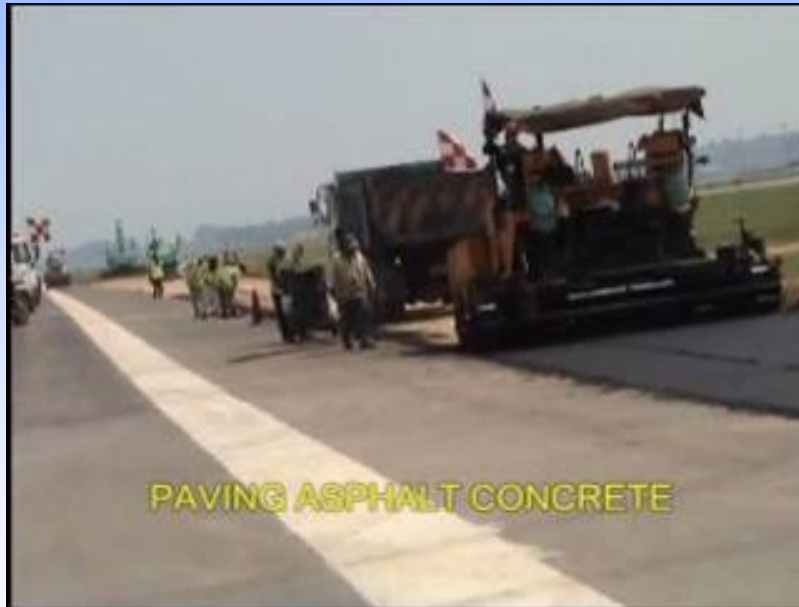
Paving Asphalt Concrete
