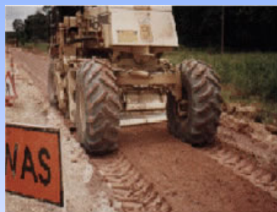
Mixing by Stabilizer
