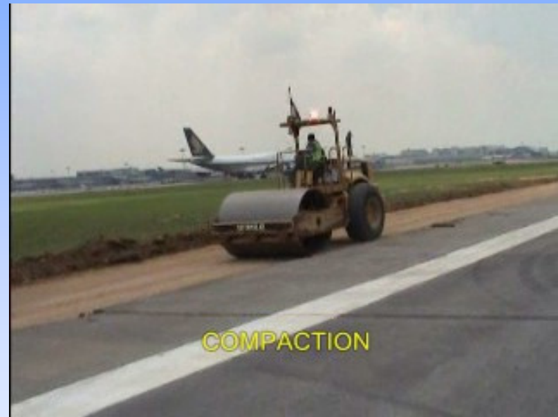
Photo 4. Compaction
