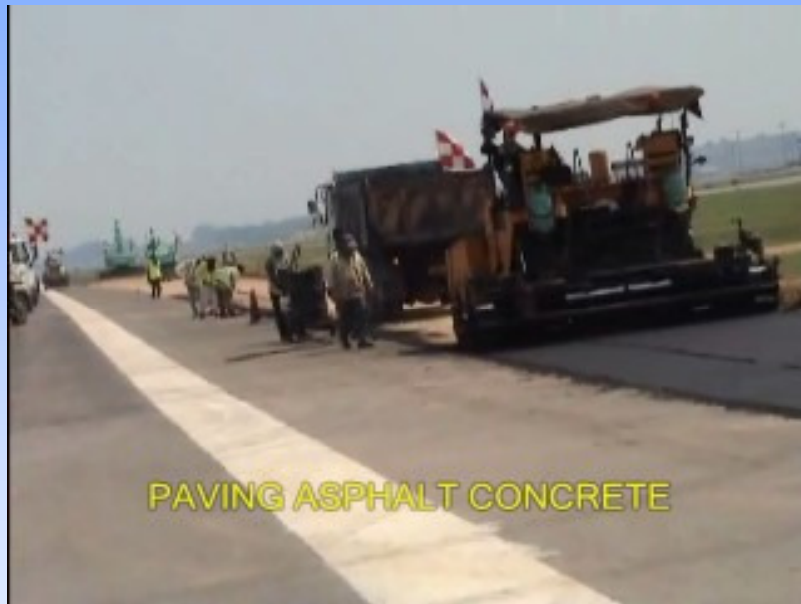
Photo 5. Paving Asphalt Concrete
