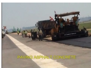
Photo 5. Paving Asphalt Concrete
