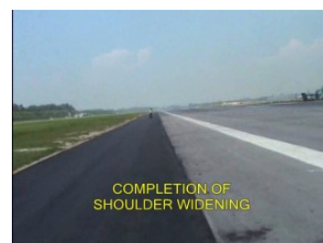
Photo 6. Completion of Widening
