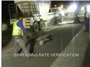
Photo 7. Spreading Rate Check
