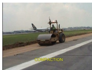
Photo 4. Compaction
