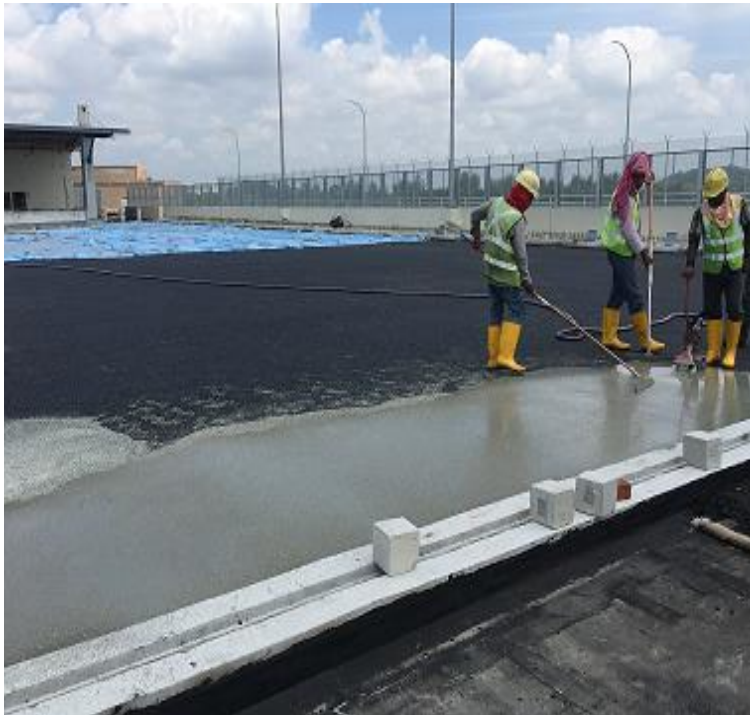
(a) Filling Grouting Material onto PAC
