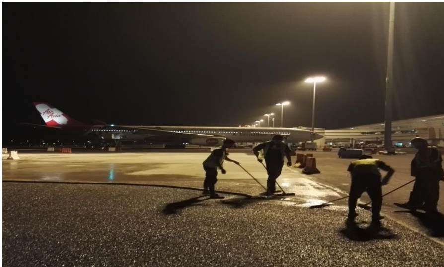
a. Laying Grouting Material
