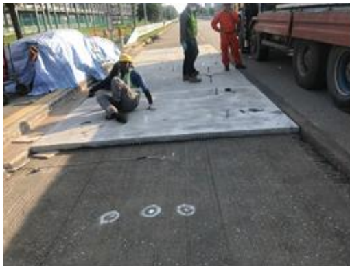
(a) Installing Precast Slab
