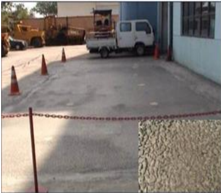
(a) Semi-Rigid Pavement after Hardened
