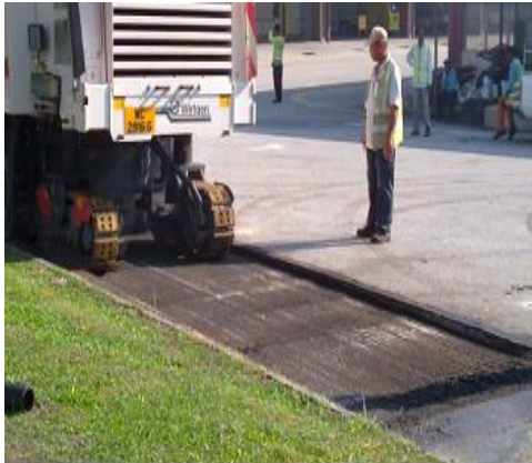
(a) Milling of Existing AC Surface
