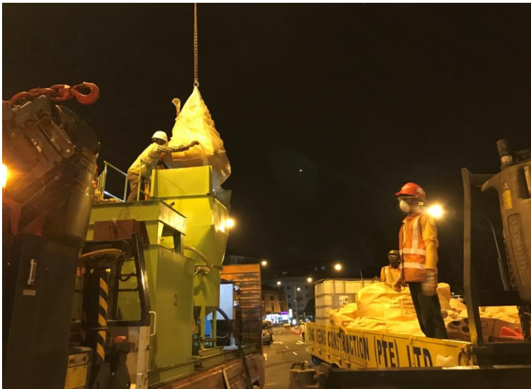
a. Mixing Grouting Material with Water
