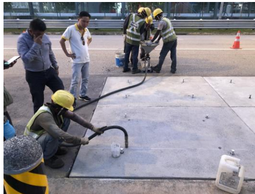
(b) Grouting for Binding
