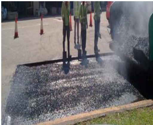
(d) Laying PAC to Designed Thickness
