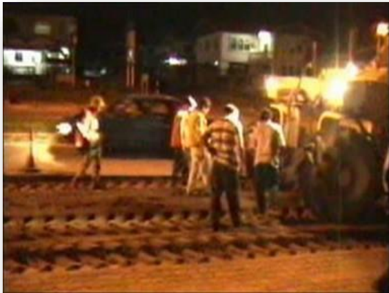
a) Rehabilitation in process
