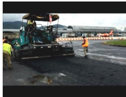
Laying of Asphalt Concrete
