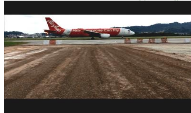
Finished Layer of Stabilized Base.
