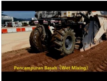
Photo 2(b)(ii) Wet Mixing
