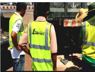
Photo 2(d)(i) In-Situ CBR Test
