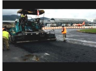
Photo 2(d)(ii) Laying of Asphalt
