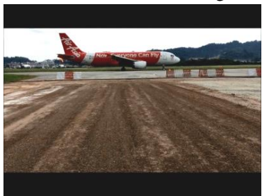
Photo 2(c)(ii) Finished Layer of Stabilized Base
