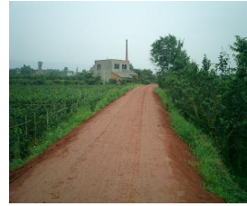
1-d Stabilized Base after Curing
