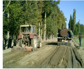
1-c Spreading & Mixing of the Liquid
