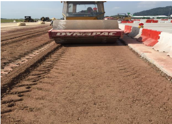
Compaction 碾压
